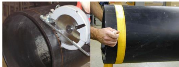
Figure IV-d – Marking and cutting larger diameter pipes
